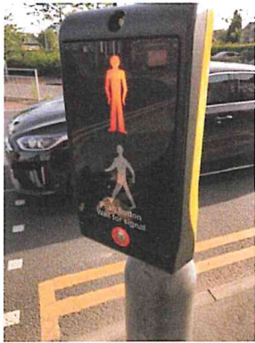
Fig 2: First Pedestrian crossing button on Middlewich Road
