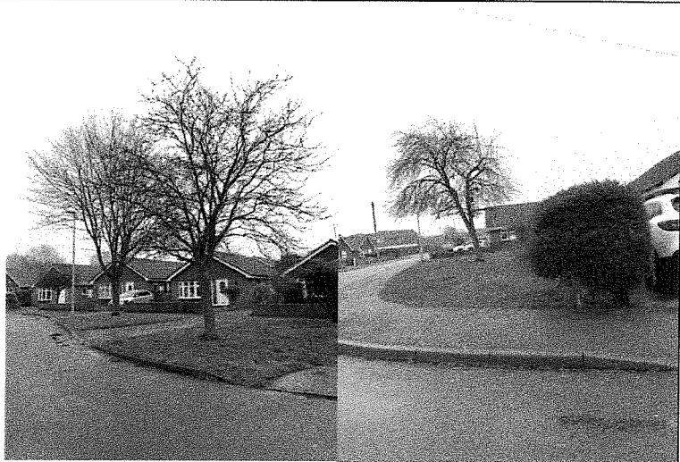
Looking south west along Gowy Close to T8 & T9 and to south down Dean Close at T10
