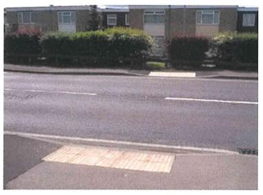
Figure 1 Example of a dropped kerb
