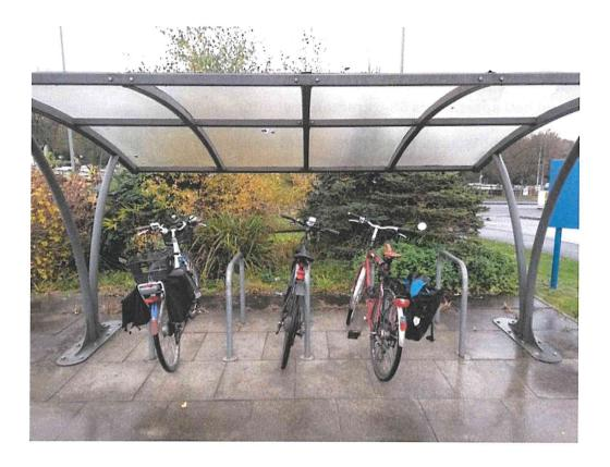
I recommend individual racks sunk into the ground as shown above, rather than a 'toast rack' (where a number of stands are fixed to 2 rails) as the bicycle wheels tend to conflict with the rails. Note, in the above example the racks are spaced too tightly. The distance between the racks must be a minimum of 1 metre, with 60 cm between the last racks in the row and the posts for the shelter, resulting in 3.20m minimum width for the shelter.
